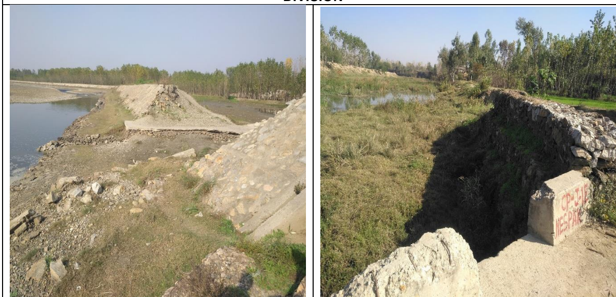
REHABILITATION OF FLOOD PROTECTION WORKS IN CHARSADDA IRRIGATION DIVISION
