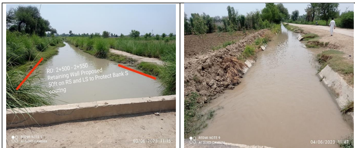
REHABILITATION OF FLOOD PROTECTION WORKS/ STRUCTURES, DIR IRRIGATION DIVISION
